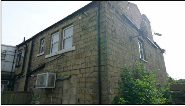
Photograph 19: South-west corner of building No.913/915
