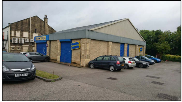
Photograph 20: South-east corner of building No.804
