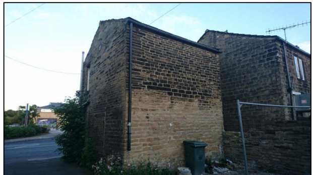
Photograph 18: Western aspect of building No.911
