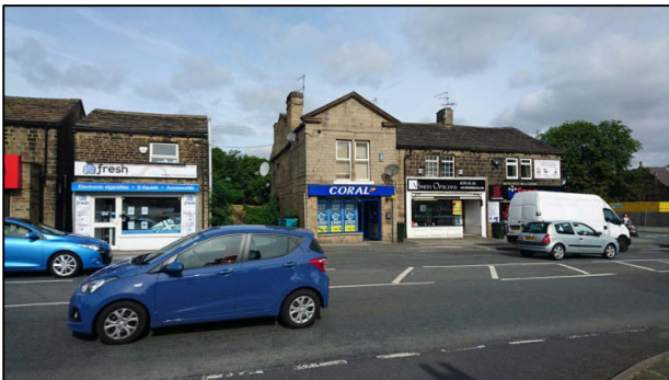
Photograph 17: Eastern aspect of buildings No.911 (left) and No. 913/ 915 (centre)
